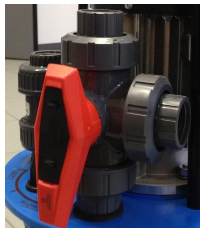
Valve in circulation position
